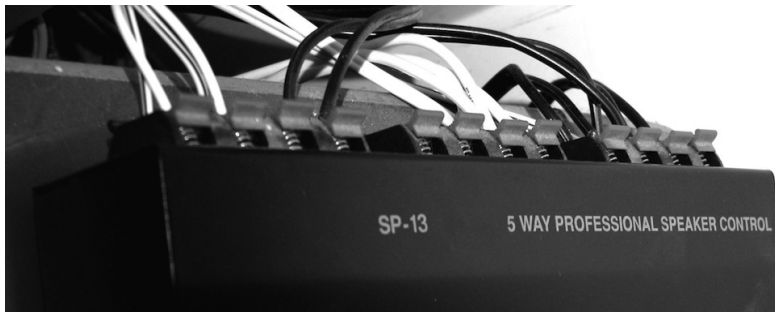
Figure 4-4. The speaker distribution bay. This model also support push-button switches to turn each speaker pair on or off (not shown).
